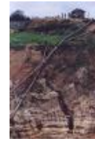
The soil and water is piped up the hill.
